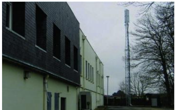
The Orange phone mast and antennas.
